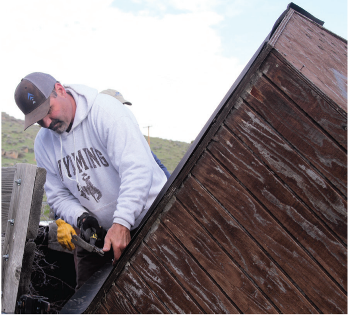
Clifford J. Smith photo Jason Marcus puts roofing paper on the top of one of the three outhouses before shingling it and finishing it off with some paint.
